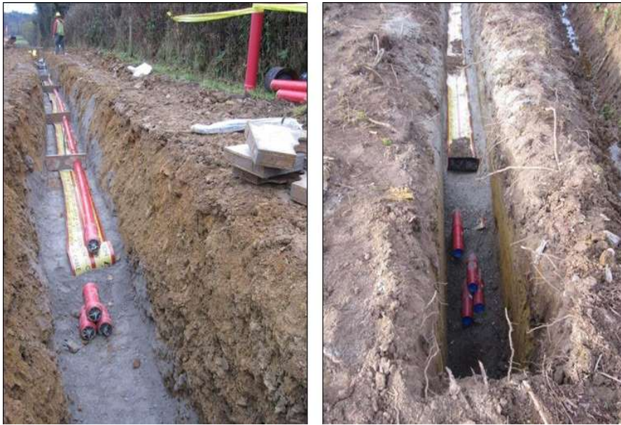
Plate 2-1 Typical Cable Trench View
